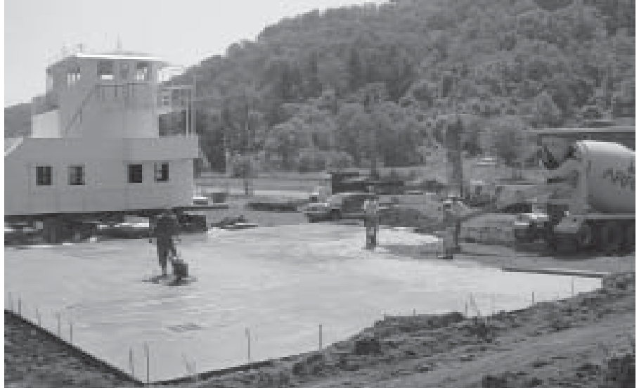
Above: RTI Research Associate John Ball, PE, designed and provided construction oversight in converting "The Warren" into a facility used to train professional, volunteer and maritime firefighters in Huntington, W.Va.
